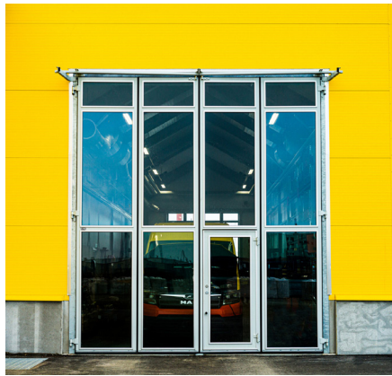
Fully glazed folding door for optimum light transmission, with recessed access door.
