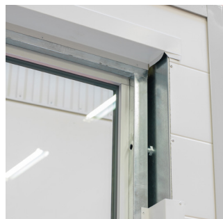
Fastening with frame screws.
