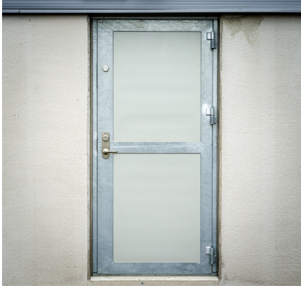
Hot-dip galvanised door leaf frame, clad with polyester lacquered sheet metal in silver metallic.
